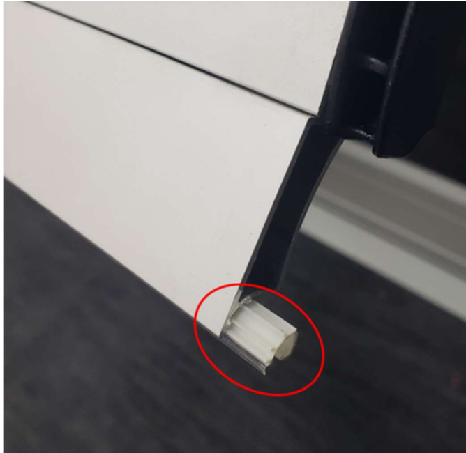
Figure 9 - Adapter lath with extruded insert in the socket
